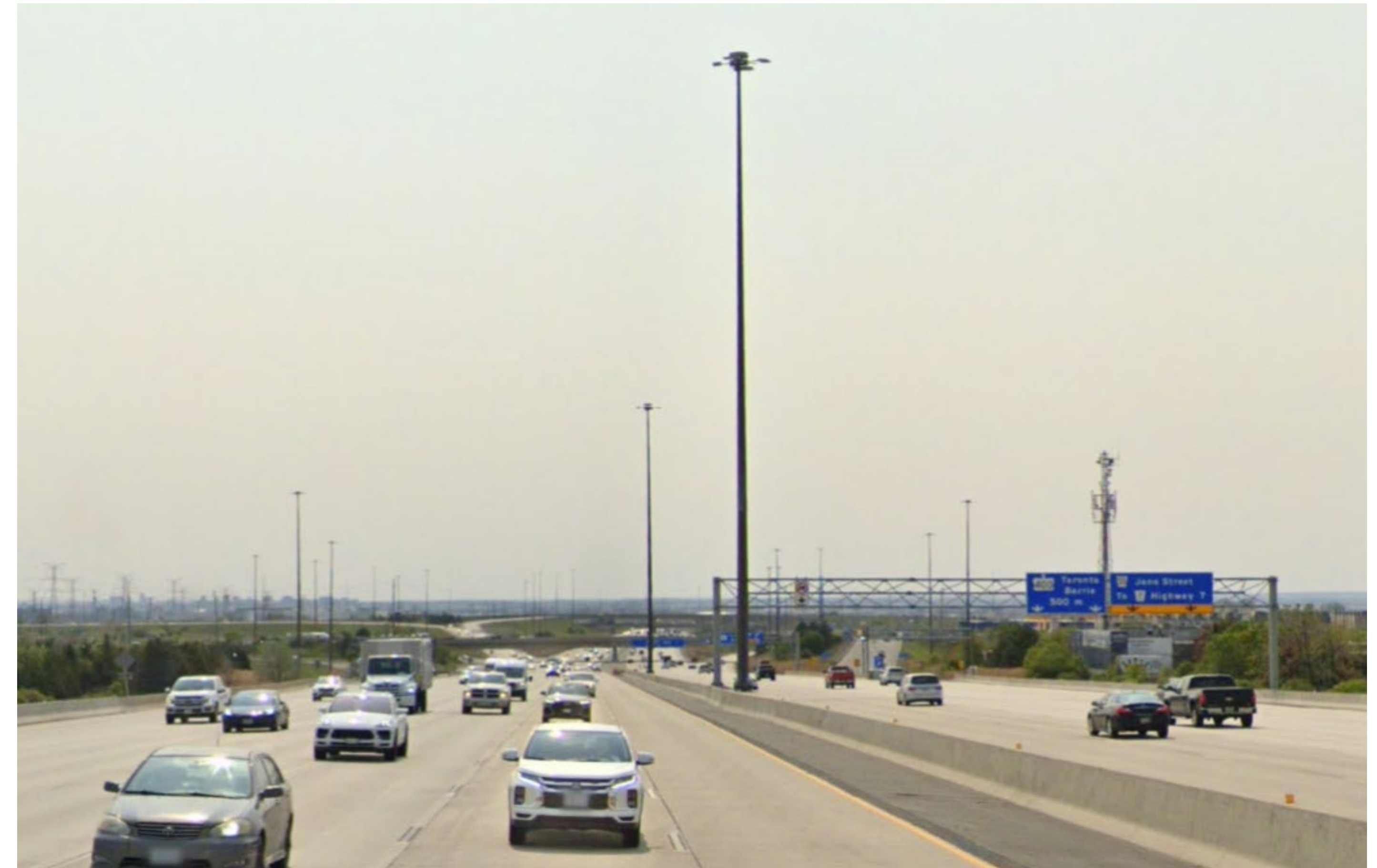
LED High Mast Lighting on Highway 407
