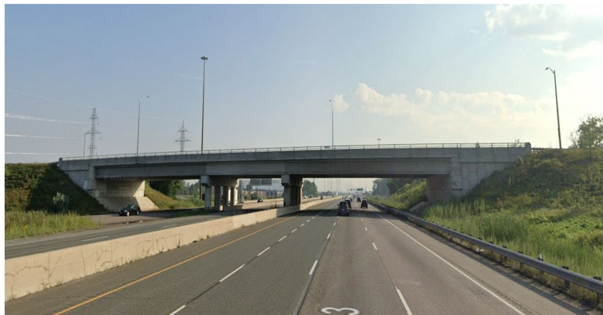
Underpass LED Lighting on Highway 403 and Ridgeway Drive
